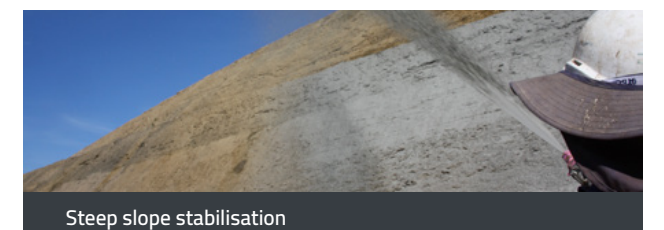
Steep slope stabilisation
