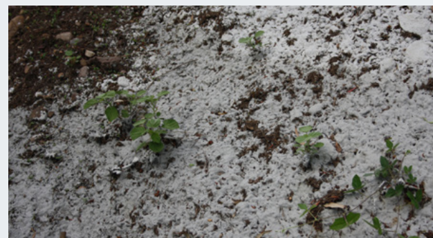
Little or no sign of delamination
